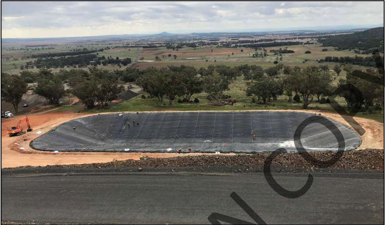
PHOTOGRAPH 2.1: Completed leachate dam. View looking north. (Source: Mackellar Excavations April 2023)
