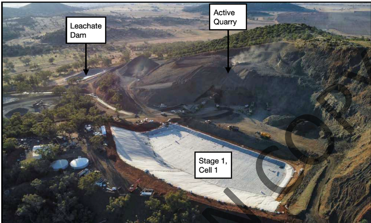
PHOTOGRAPH 1.1: View of completed Stage 1 Cell 1, quarry and Leachate Dam
